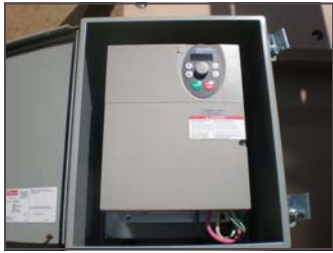
Electronics Enclosure housing the variable frequency drive system
